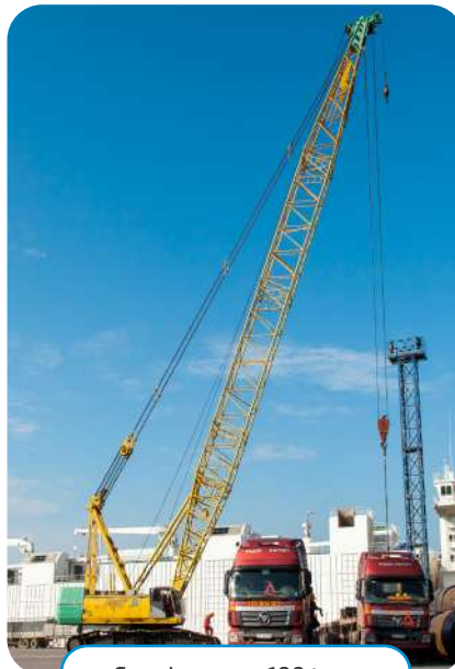
Crawler crane 100 tons
