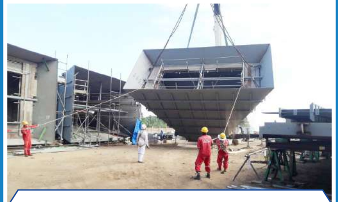
Hopper Fabrication – Long Phu Thermal Power Plant
