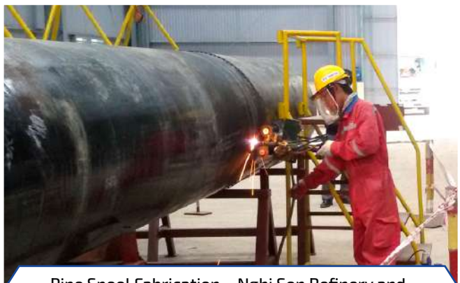
Pipe Spool Fabrication – Nghi Son Refinery and Petrochemical Project
