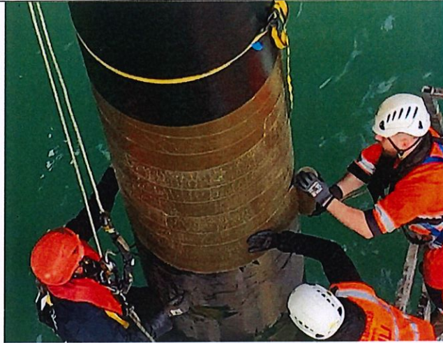
Figure 5. Apply Petrolatum Wrapping Tape
