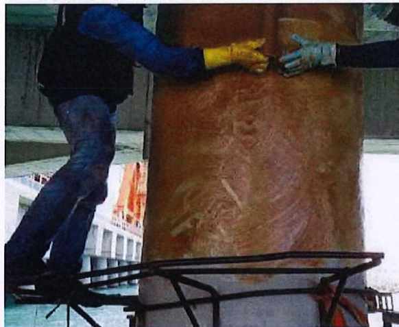
Figure 4. Layers apply for protection Pile
