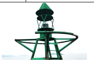
The insurant brim is broken
